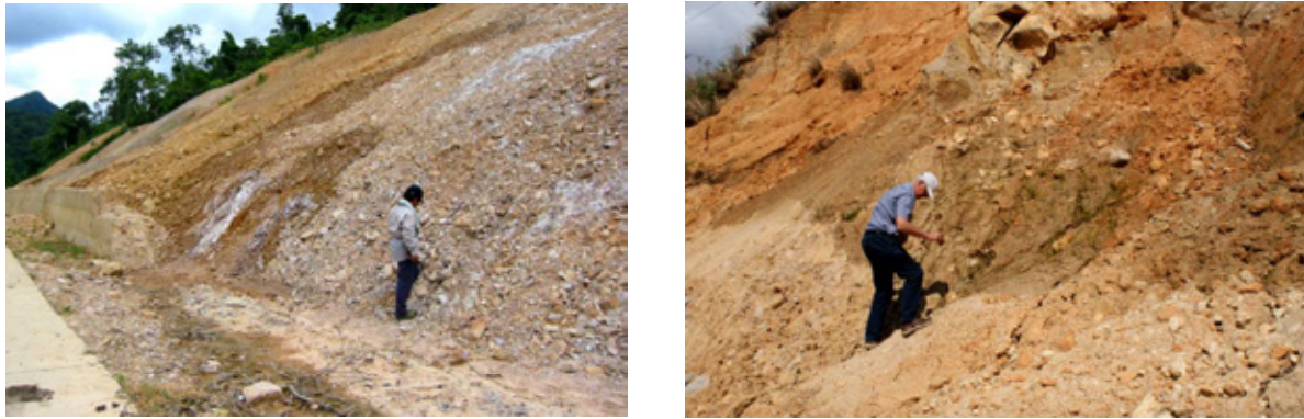
Fig.37. Improper drainage is an important cause of slope failure: Left photo taken in 8/2004 at Deo Da Deo Pass (Quang Binh province) at the beginning of the rainy season; Right photo taken in 4/2011 at Deo Sa Mui Pass (Quang Tri province) during the dry season
