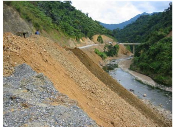
Fig.29. Improper rock/soil waste disposal which will be washed very far downstream
