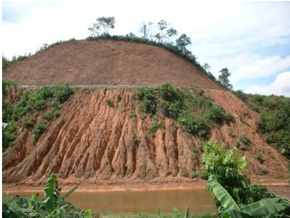
Fig.29. Improper rock/soil waste disposal which will be washed very far downstream
