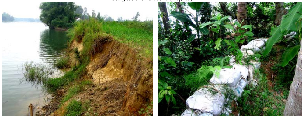
Fig.4. Another section of the poorly eroded bank at Binh Thoi Commune, Tra Khuc River (left) and the traditional, primitive protection by local farmers using sand bag (right)
