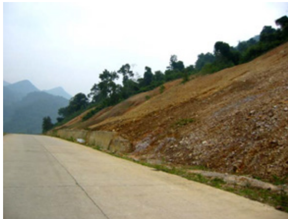
Fig.33. Without Vetiver grass, the slope constructed out on strongly crushed rock/soil along a fault zone at Deo Da Deo Pass (Quang Binh province) continuously fails even though it has been very gently flattened down to the natural slope angle (photos taken 8/2004)
