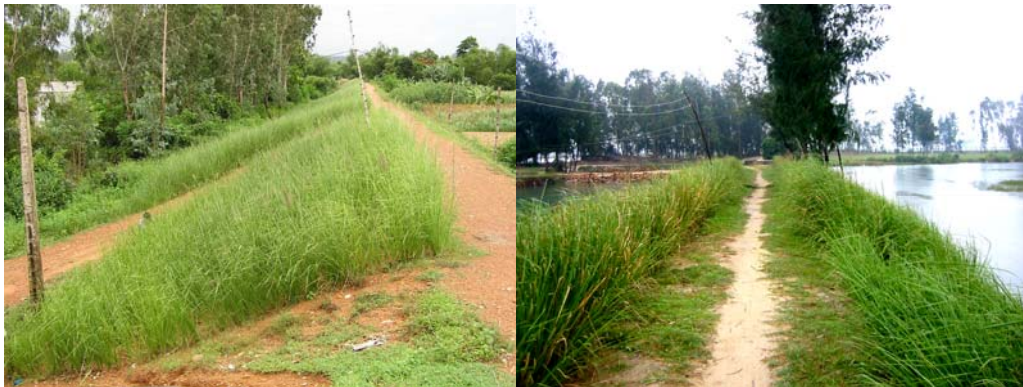
Fig.2. Left: Vetiver grass planted on river dike along Tra Bong River; right: on both sides of an anti-salinity estuary dike along the same river
