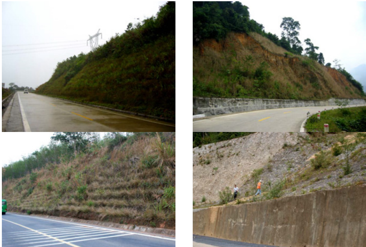
Fig.40. As Vetiver is seasonal and no longer maintained, local, perennial species strongly come back to compete, penetrating even the rock rip-rap and wire mesh (lowermost photo, taken 4/2011)
