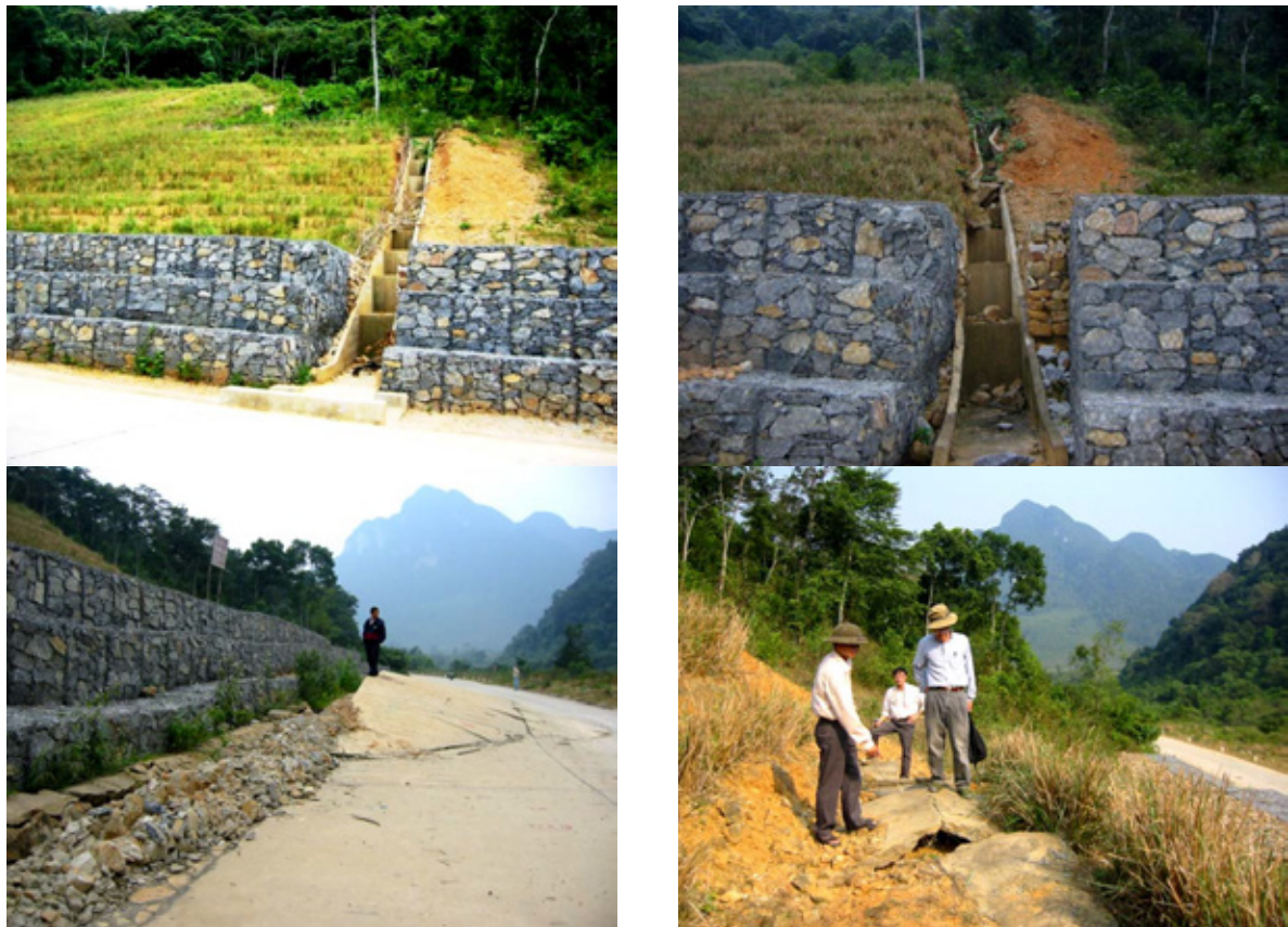
Fig.35. (Same location). Planted just in 6/2004 (left photo taken 8/2004), the grass couldn't help prevent a deep failure in 9/2004 during the rainy season (right photo taken 1/2005)
