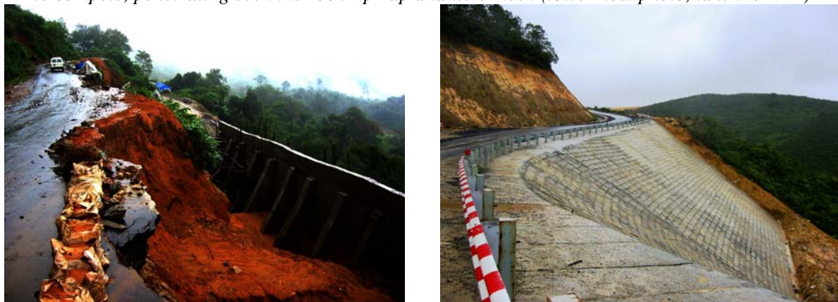
Fig.41. Failure of the negative side of cut slopes and rigorous remedial measures
