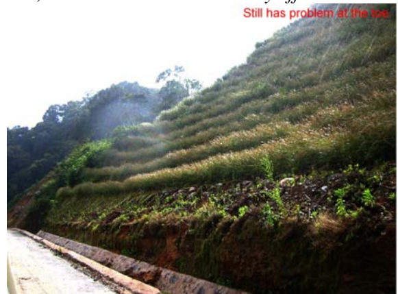
Fig.31. Protection of the slope toe is a must to ensure stability
