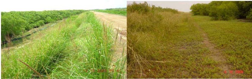
Fig.8. Planting Vetiver grass in Go Cong province, behind the natural mangrove on this Acid Sulfate Soil sea dike. Surface erosion is reduced and local grass re-established
