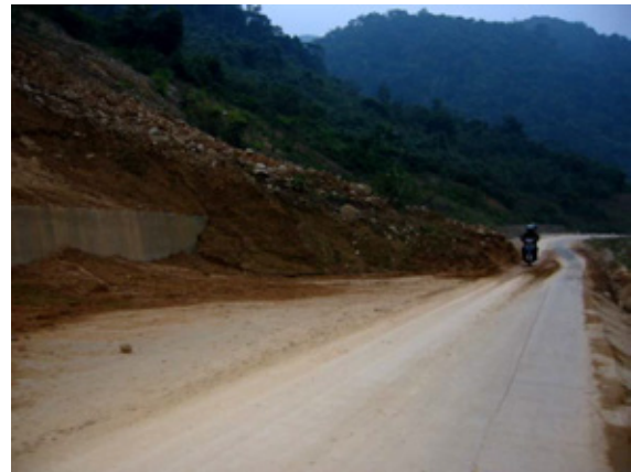
Fig.33. Without Vetiver grass, the slope constructed out on strongly crushed rock/soil along a fault zone at Deo Da Deo Pass (Quang Binh province) continuously fails even though it has been very gently flattened down to the natural slope angle (photos taken 8/2004)
