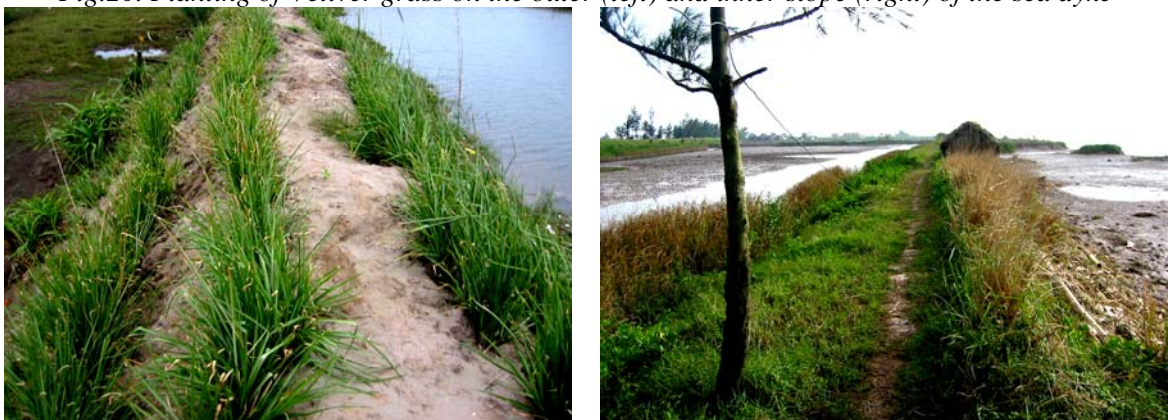
Fig.21. Planting of Vetiver grass on anti-salinity dyke
