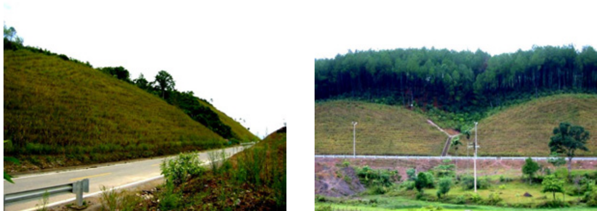
Fig.38. With proper design, Vetiver rows can help greatly divert the surface run-off, reduce infiltration and stabilize the slopes (photos taken in 8/2004 in Vu Quang, Ha Tinh province)
