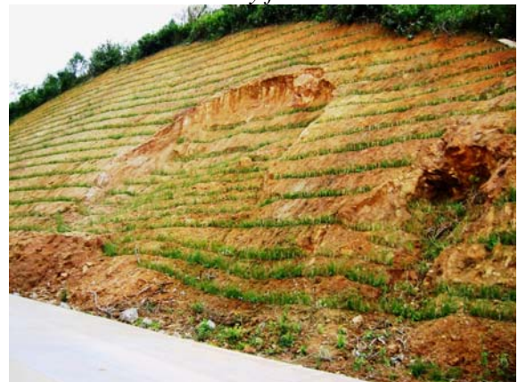
Fig.30. The slopes should first be internally stable, as the VS is not immediately effective
