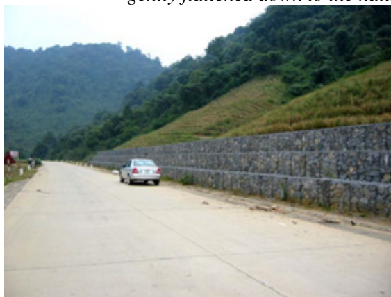
Fig.34. Under the same condition, a combination of Vetiver grass and rock groins did a better job even though at the other end still couldn't prevent a massive failure to occur (photos taken 1/2005)
