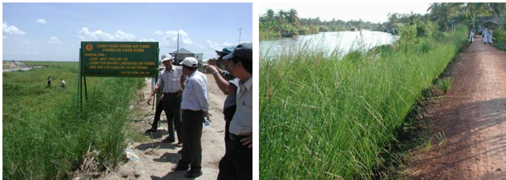
Fig.6. Vetiver grass and river dike (left) and along a natural river bank (right) in An Giang
