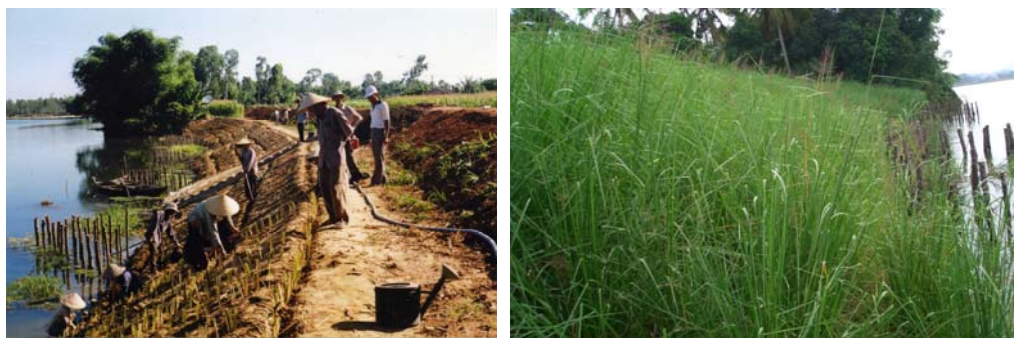
Fig.5. Vetiver grass comes in with local participation (left) and the bank stays intact after the flood season in Nov. 2005
