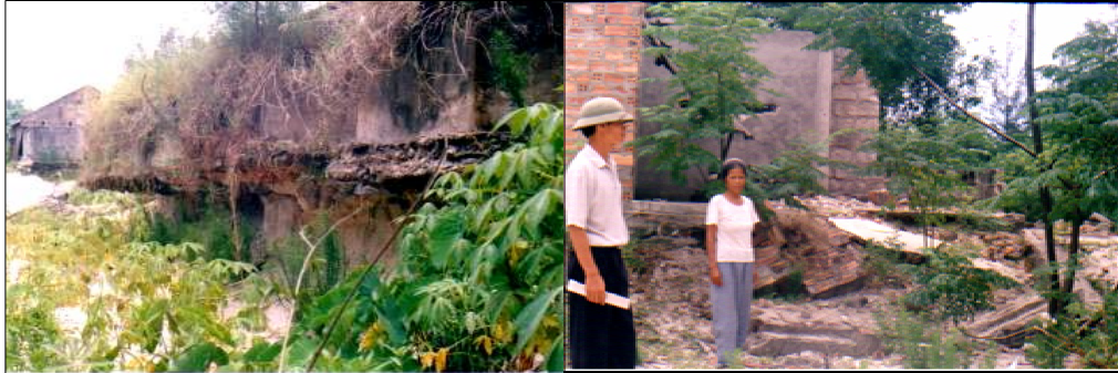
Fig.1. Sand flow in Le Thuy (Quang Binh) in 1999, exposing the foundation of a pumping station (left) and a 3-room brick house (right)
