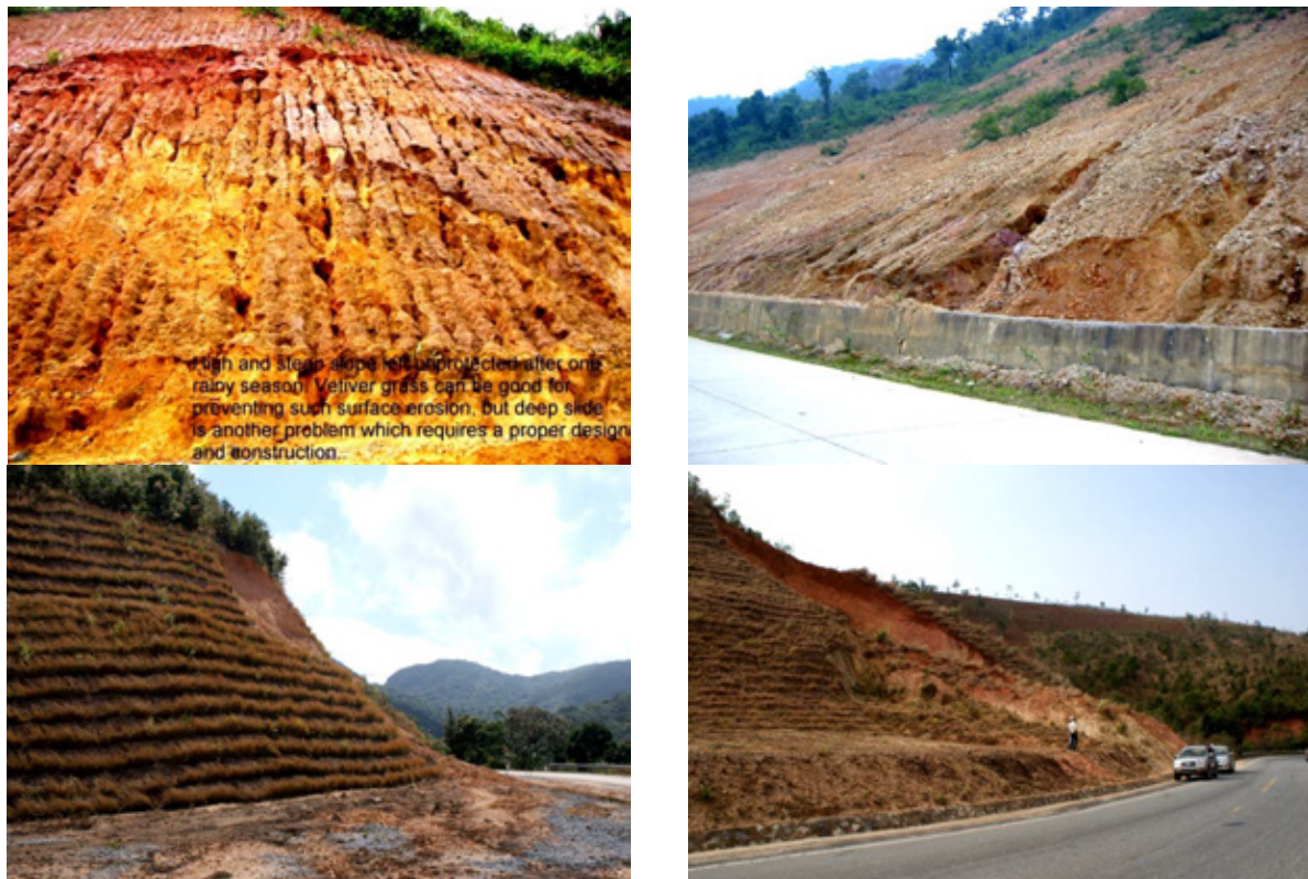
Fig.32. Slope surface erosion, developing into gullies and small, shallow landslides before large, deep-seated ones take place and Vetiver grass cannot help
