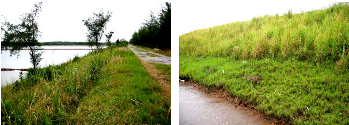
Fig.20. Planting of Vetiver grass on the outer (left) and inner slope (right) of the sea dyke
