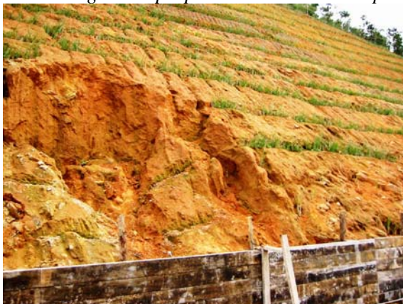
Fig.30. The slopes should first be internally stable, as the VS is not immediately effective
