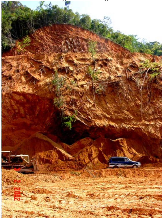
Fig.25. Many cut slopes designed and constructed not to the standard, tens of m in height, very steep, often >60-75° with rare or even without benches etc.
