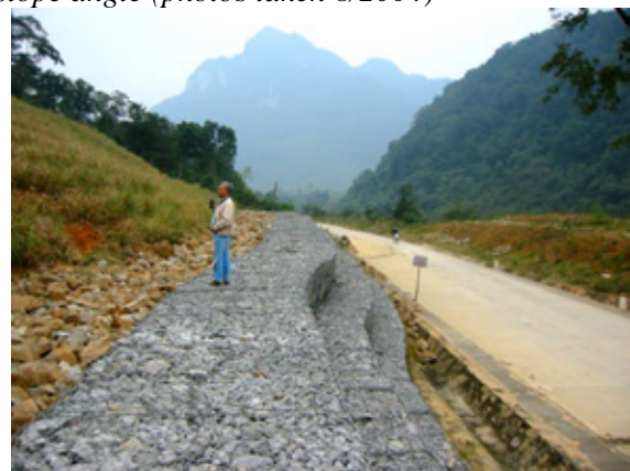
Fig.34. Under the same condition, a combination of Vetiver grass and rock groins did a better job even though at the other end still couldn't prevent a massive failure to occur (photos taken 1/2005)
